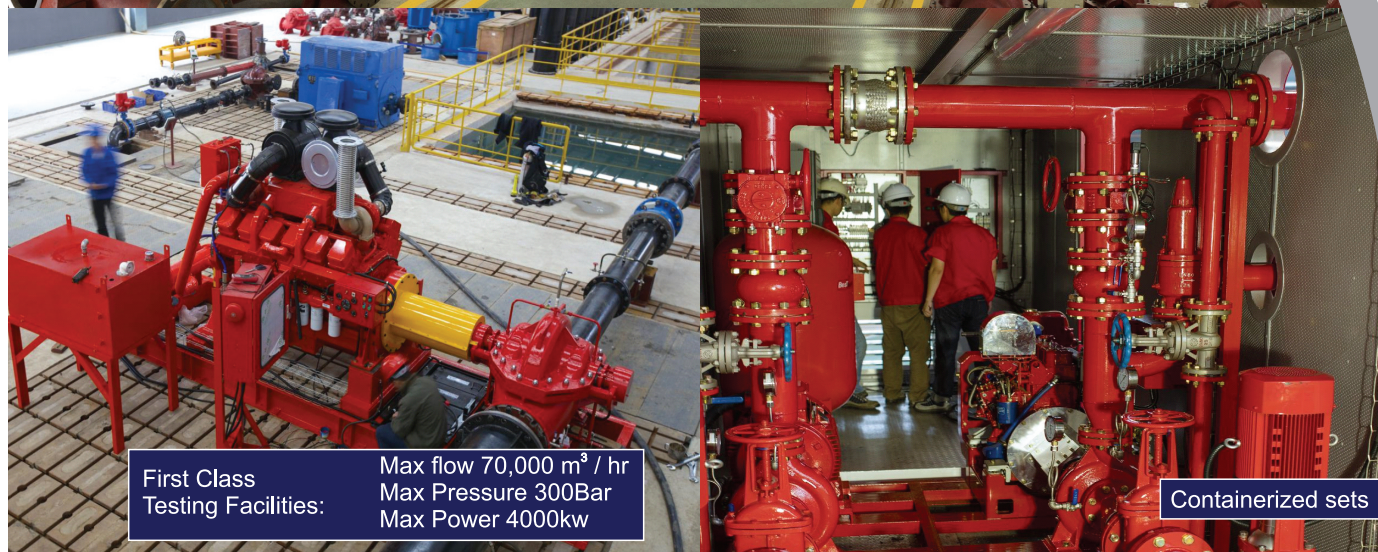
50 000 m 2 Fire Facility
